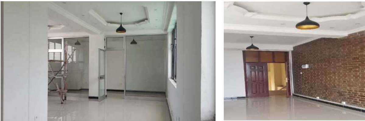
Figure 9 CDT-Africa Innocafe at final stages of renovation
